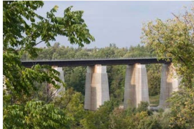
GTR Viaduct, Georgetown
